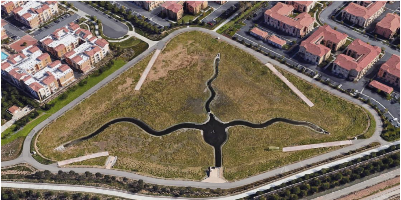
Typical Detention Multi-Benefit Trash Treatment System
