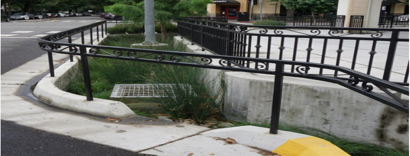
Figure A: Urban Infiltration Trench
