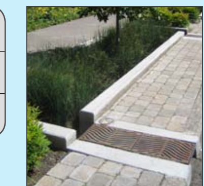
An overflow outlet conveys runoff that exceeds the bioretention area capacity.
