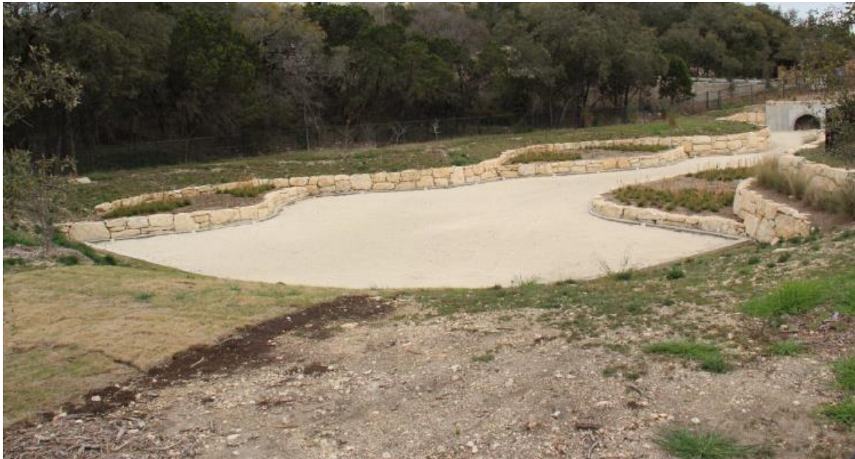
Figure A: Media Filter BMP Image - County of San Diego LID Handbook
