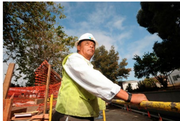
San Leandro Creek floodwall construction
