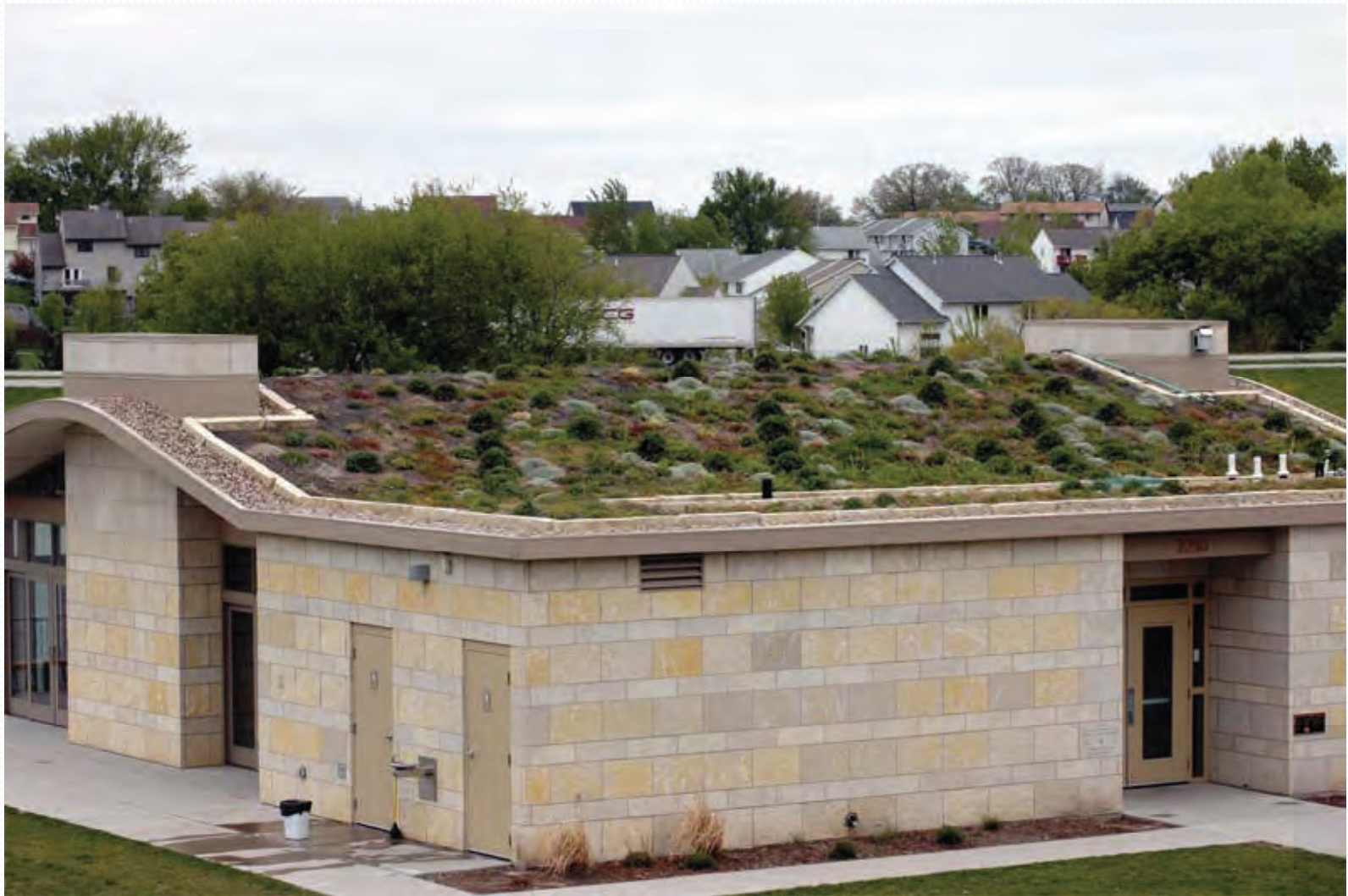
Park Building, Coraville, Iowa. Photo courtesy of NRCS
