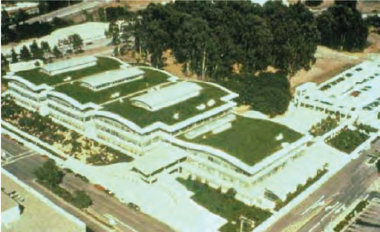
Green Roof (Gap Headquarters – San Bruno)
