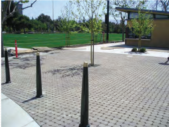
Permeable Pavers, Palo Alto/Stanford Community Playing Fields
