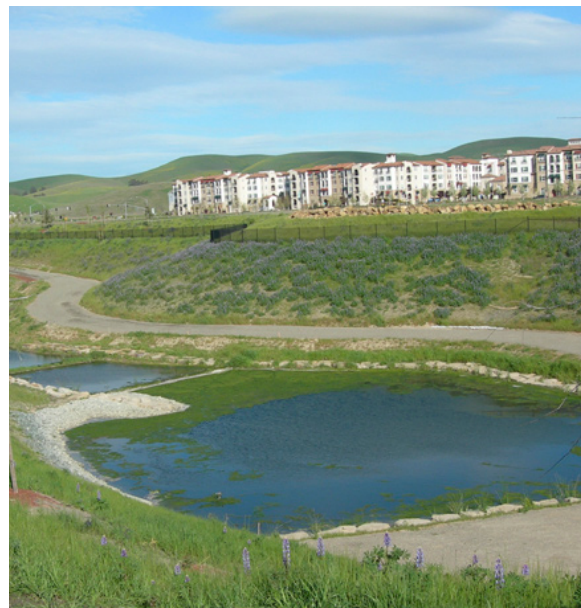
Presentation on TMDL (left); Water quality basin in Dublin, designed to hold low-flow stormwater runoff (right)
