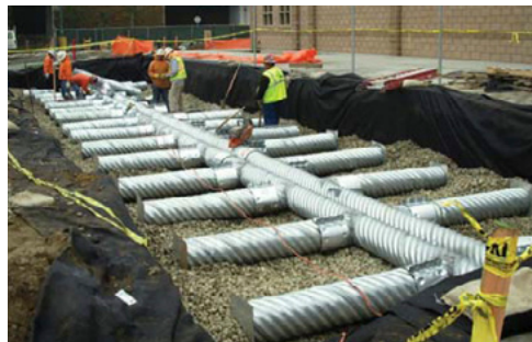
Disneyland Resort (top) and a view of the resort's Central Bakery stormwater infiltration system components during construction (above)
