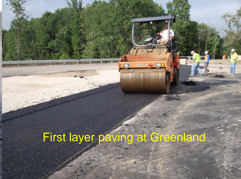
First layer paving at Greenland
