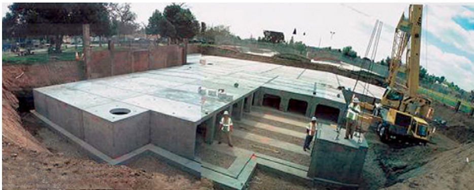
Construction of the below-ground water treatment facility at Garvanza Park in Los Angeles (left); Project features such as storm drains, sedimentation, retention and settling basins, pre-treatment systems and infiltration gallery (right)
