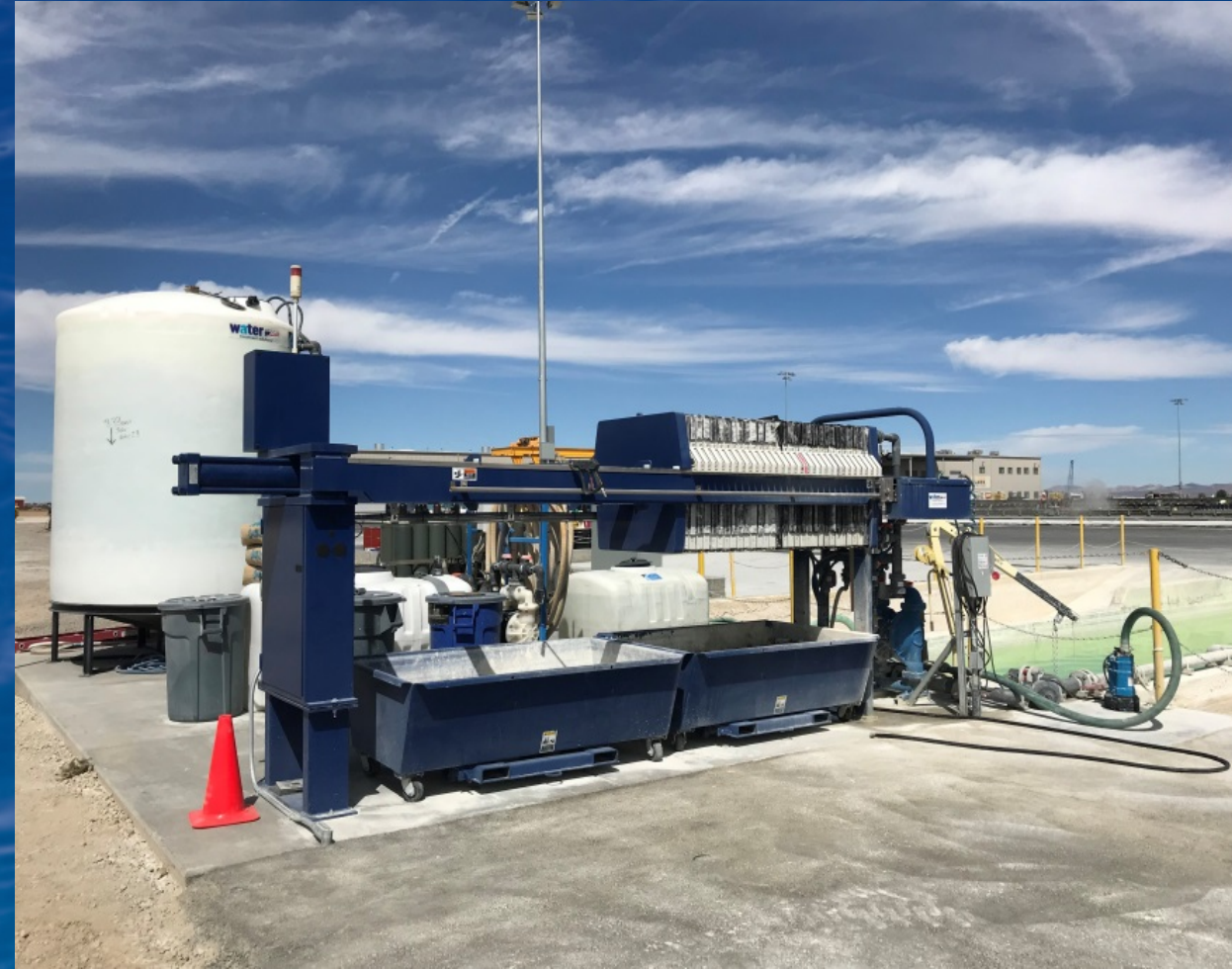
Process Water Recycling Ponds
