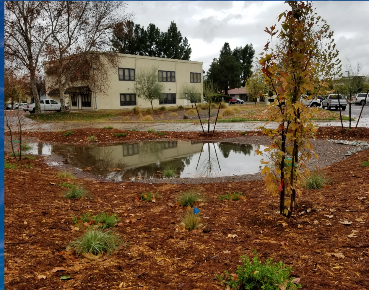
Runoff Capture and Infiltration Basin
