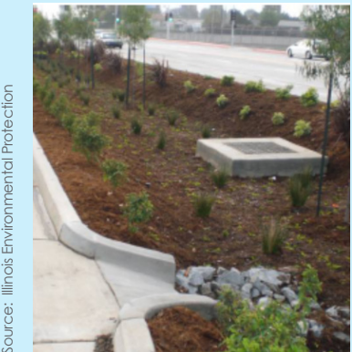
An overflow outlet conveys runoff that exceeds the bioretention area capacity.
