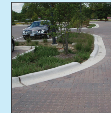
A curb cut inlet directs stormwater runoff into a biofiltration planter.
