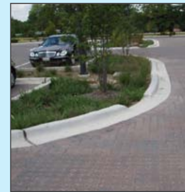
A curb cut inlet directs stormwater runoff into a biofiltration planter.
