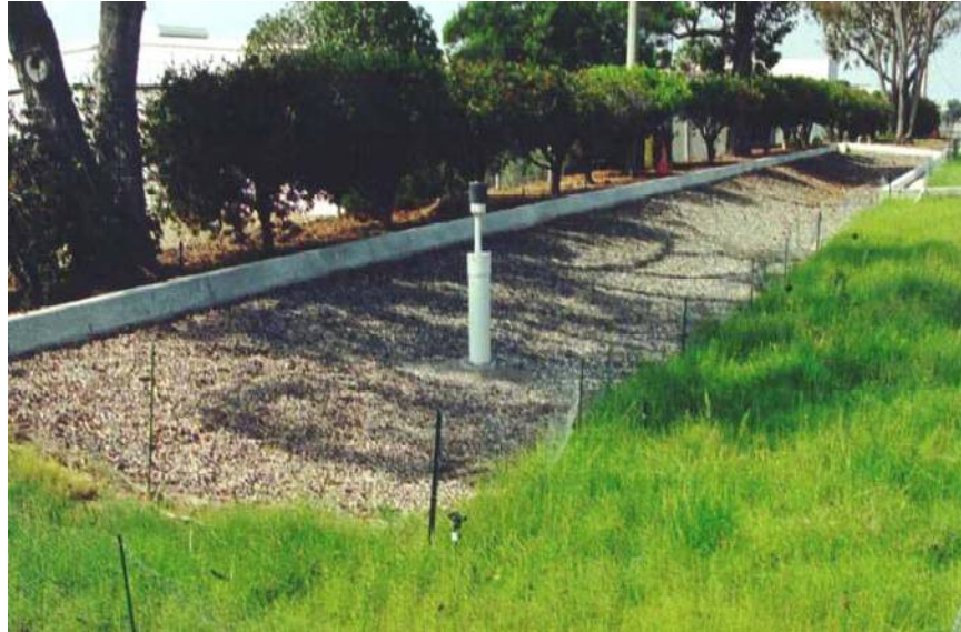
Figure 78. Infiltration Trench. Source: RBF Consulting
