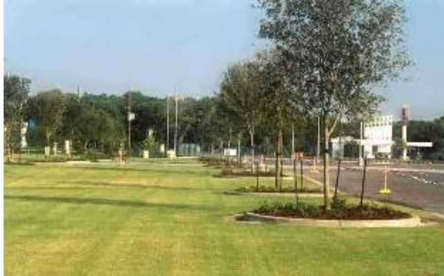
Figure 53. Reinforced turf used as overflow parking area. Source: Cahill Associates
