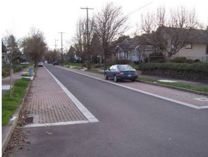
Figure 38. Pervious paver parking edge in residential neighborhood in Portland Oregon. Source: Cahill Associates
