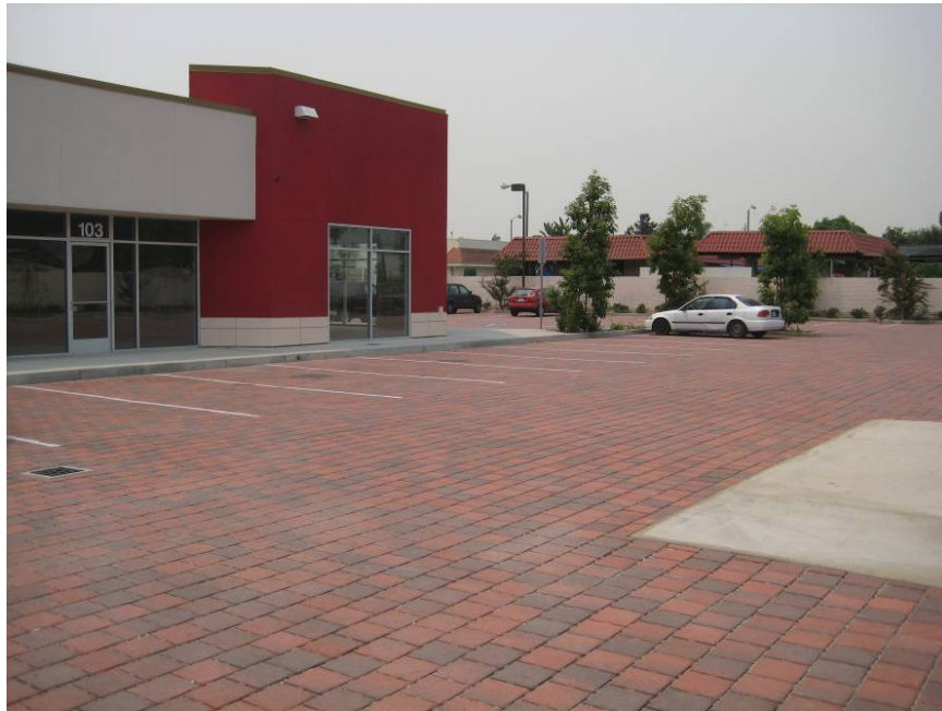
Figure 32. Parking Lot, City of Downey, CA. Source: California Watershed Engineering
