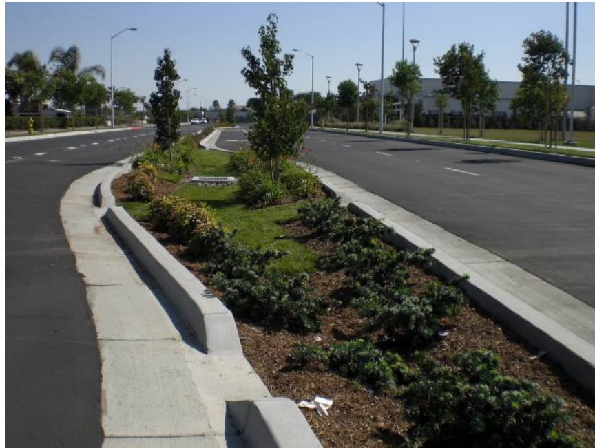
Figure 24. Bioretention cell for street/yard drainage, Downey, CA.
