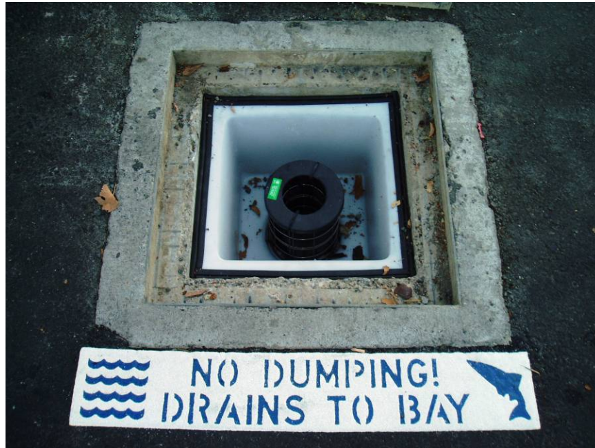
Figure 83. Catch basin insert. Source: REM Inc.
