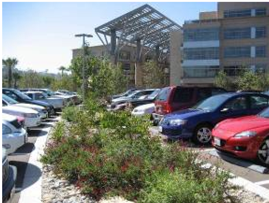
Figure 17. Bioretention Cell in Parking Lot, Caltrans District 11 Headquarters, San Diego, CA. Source: Wallace Roberts & Todd, Inc.
