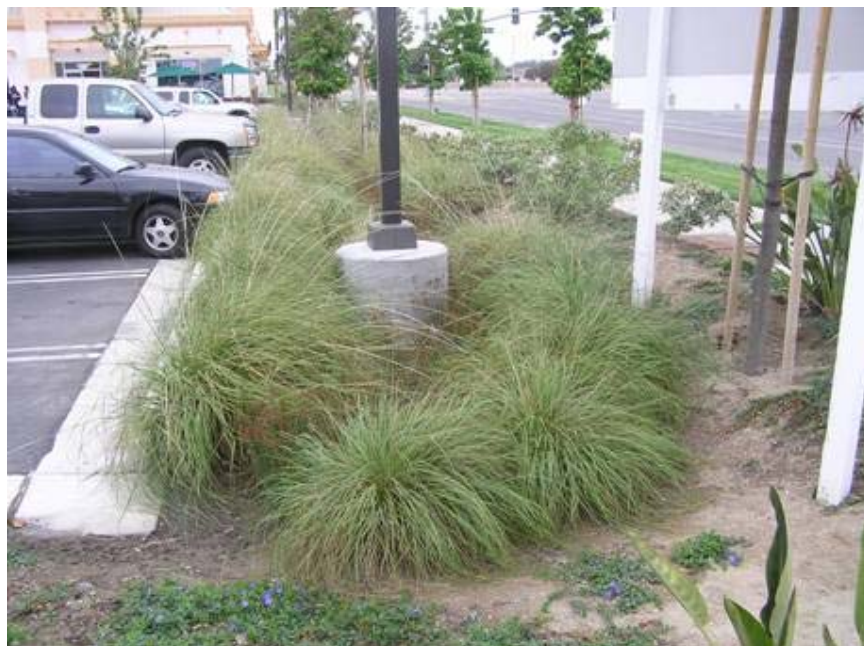
Figure 21. Parking Lot Bioswale, Oxnard, CA. Source: Ed Gripp
