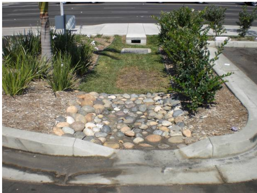
Figure 27. Inlet Structure, Downey, CA. Source: Bill DePoto
