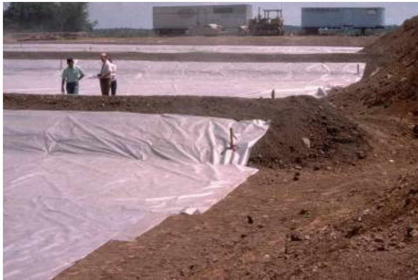
Figure 57. Earthen berms separate terraced infiltration beds. Source: Cahill Associates
