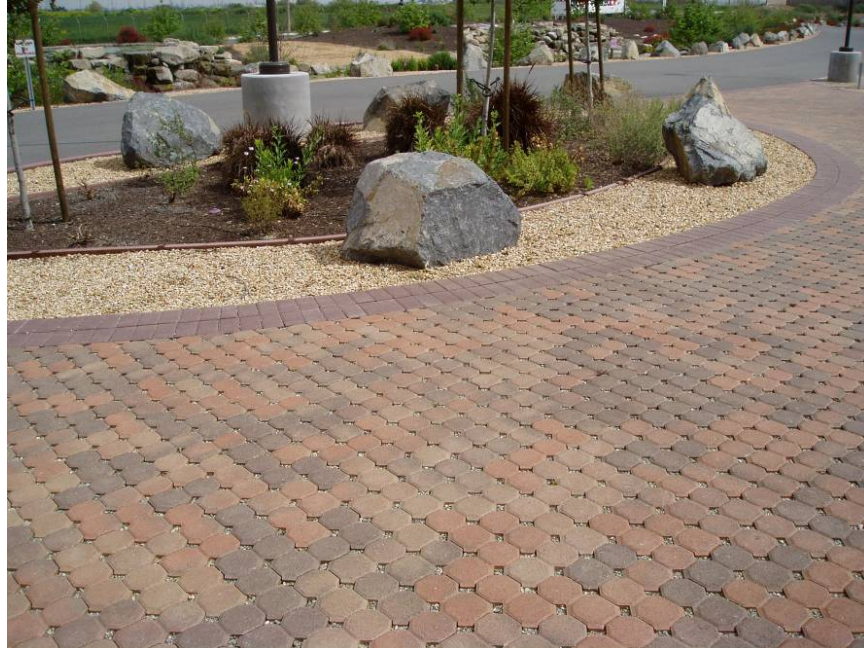
Figure 34. Pervious Paver Driveway, Chino, CA. Source: Jeff Endicott
