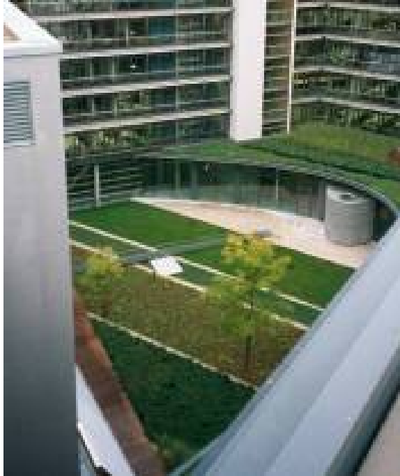
Figure 64. Large cistern for vegetated roof plaza maintenance. Source: Cahill Associates
