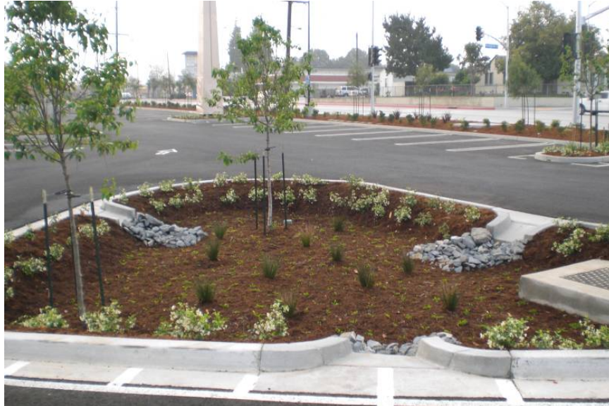
Figure 29. Newly Planted Bioretention Cell in El Monte, CA. Source: Bill DePoto
