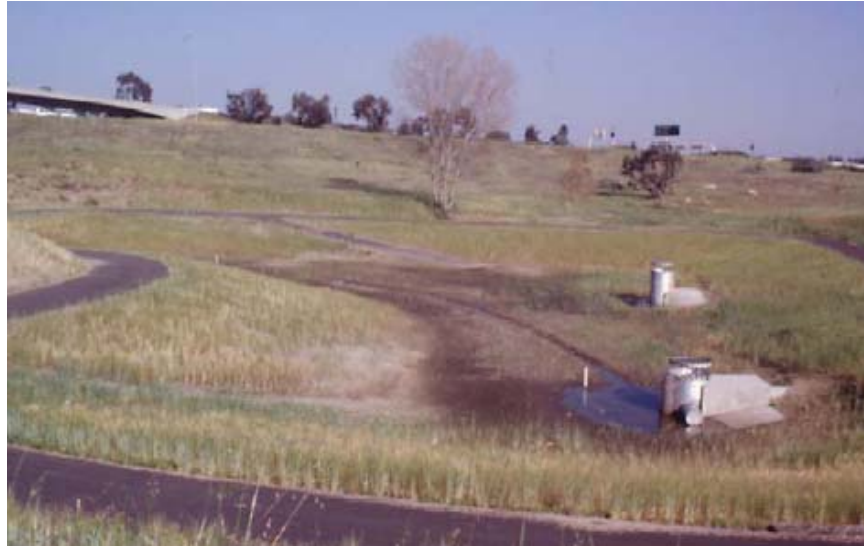
Figure 80. Dry pond. Source: RBF Consulting
