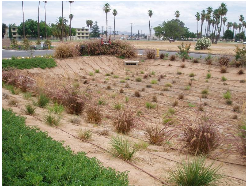
Figure 77. Infiltration Basin. Source: March Joint Powers Authority
