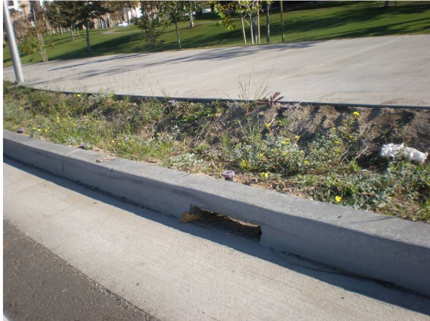
Figure 75. A vegetated swale with curb cuts in Playa Vista, California. Source: Keith Linker
