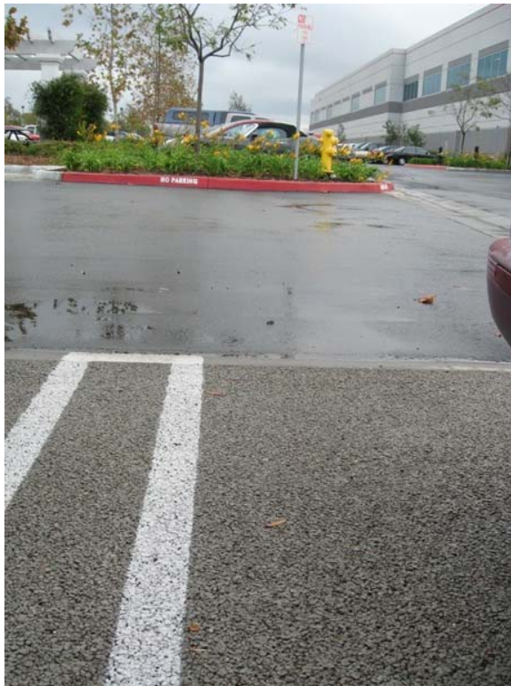
Figure 43. Pervious concrete parking areas, Haas Automation, Inc., Oxnard, CA. Source: Lorraine Rubin
