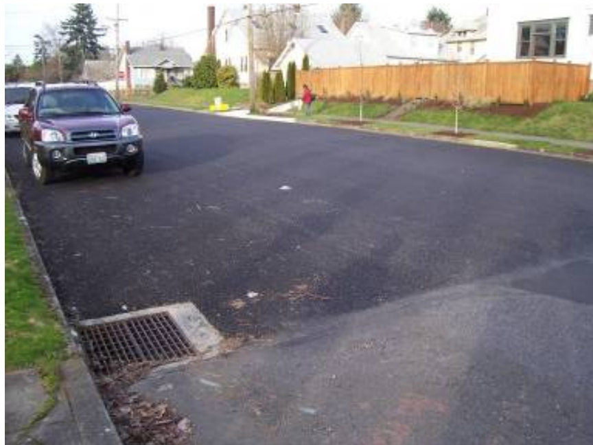
Figure 37. Pervious asphalt street in residential neighborhood in Portland Oregon. Source: Cahill Associates
