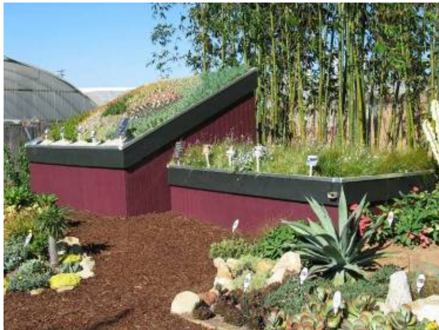
Figure 68. Demonstration vegetated roof project at EuroAmerican Growers in Bonsall, CA. Source: Technical Advisory Committee
