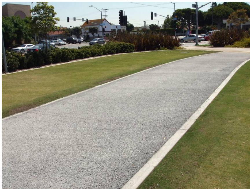
Figure 35. Pervious Concrete Sidewalk, Santa Monica, CA. Source: Bill DePoto
