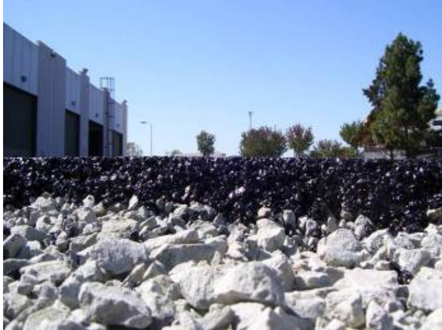
Figure 41. Close-up showing pervious asphalt pavement atop a stone infiltration/storage bed at the San Diego County Operations Center in Kearny Mesa, CA.
