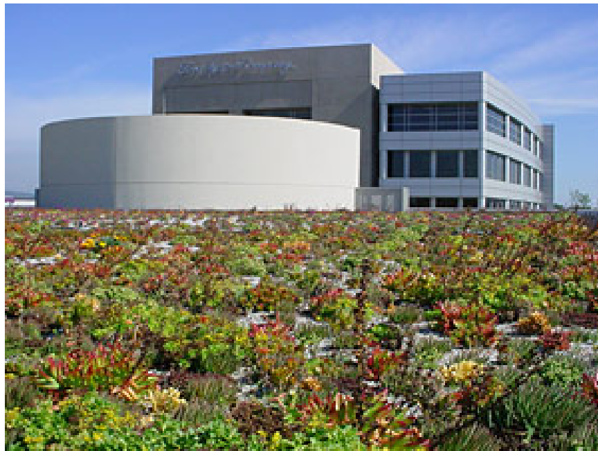
Figure 70. Premier Automotive Headquarters, Irvine. Source: Roofscapes, Inc.
