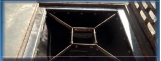
DrainPac™ Filter Insert – Retains pollutants inside filter basket
