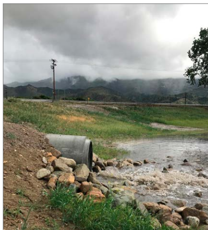
Outfall and stormwater discharge onto Piru Spreading Grounds
