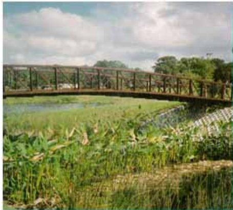
Figure 1. Constructed wetland (EPA)
