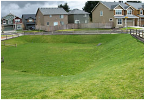
Figure 1. Extended Detention basin (Stormwater Partners SW Washington)
