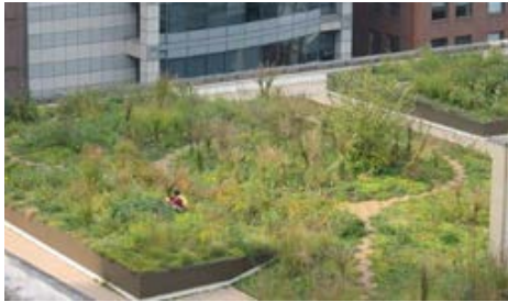
Figure 1. Green roof (Center for Neighborhood Technology)
