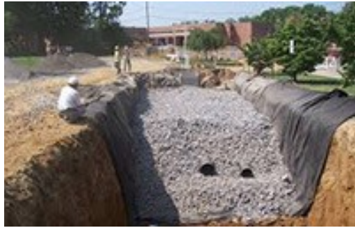
Figure 1. Infiltration trench (Richland Soil and Water Conservation)
