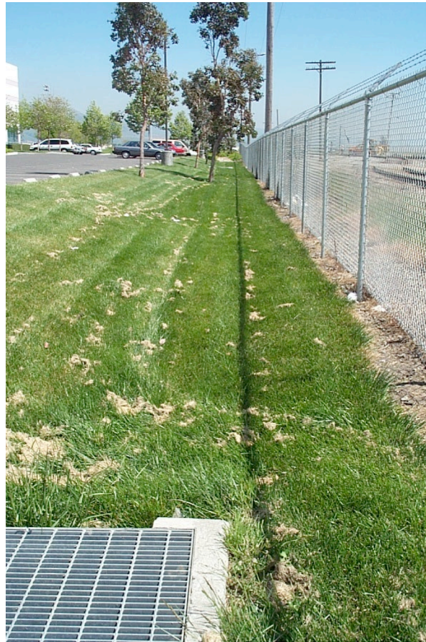
A grassy swale treats the runoff from this galvanized fence
