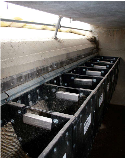
Photo 3: Curb Inlet Install with Multiple Units
