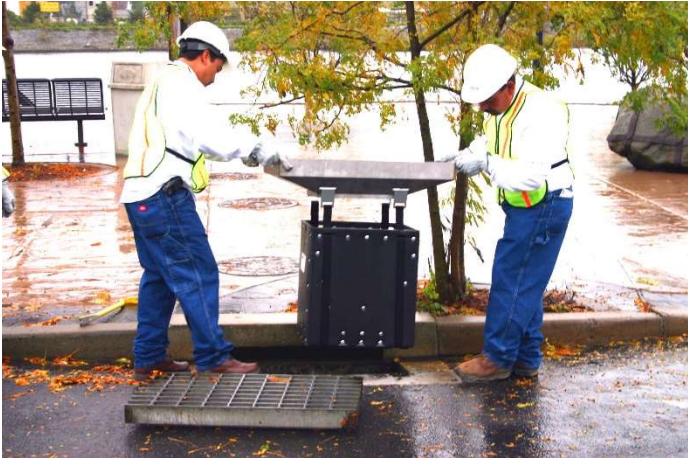
Photo 1: Drop-In UUF Install with two man team
