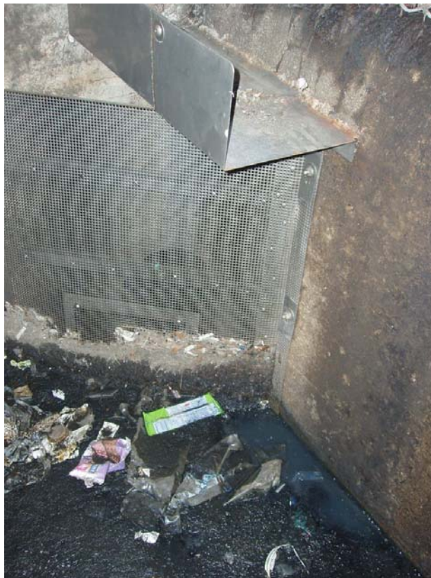
Figure 10. Rectangular screen across CB corner
