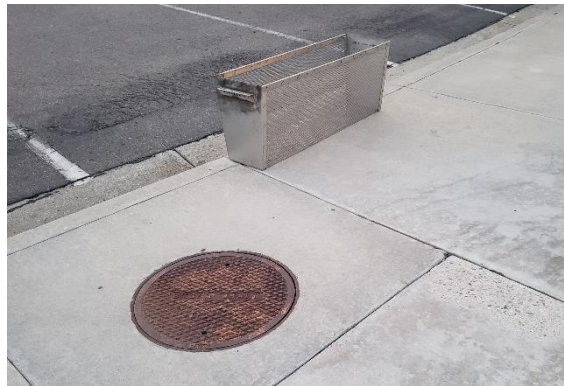
Figure 8 - Curb Inlet Filter Being Installed.
