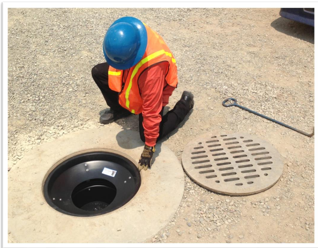
Image 9: Installation of a unit.
