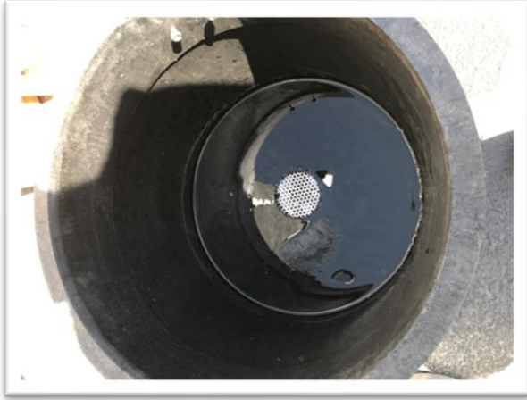
Image 13: 3/16" Screen at 3 inch diameter opening.
