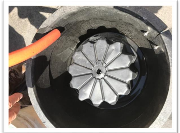
Image 14: Energy Dissipater added to top of opening to avoid jet flow.
