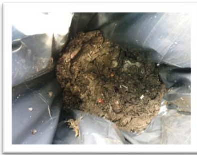
Image 11: Inspection and Cleaning of a side inlet with a Water Decontaminator Model #TCU-4. Leaves and sediment present and removed. Housing cleaned, sediment collected and disposed. Note special support frame. ( Deflector removed for visual purposes )
