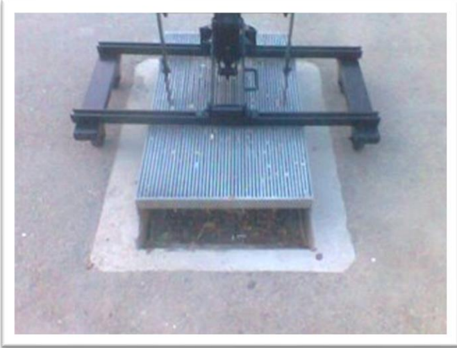
Image 8: Lifting of grate in a parking lot with a special lifting mechanism.
