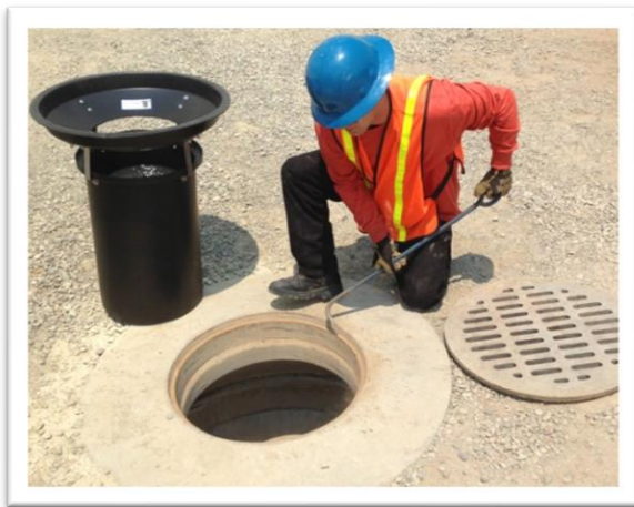
Image 6: Installing unit, checking lip and removing rust.
