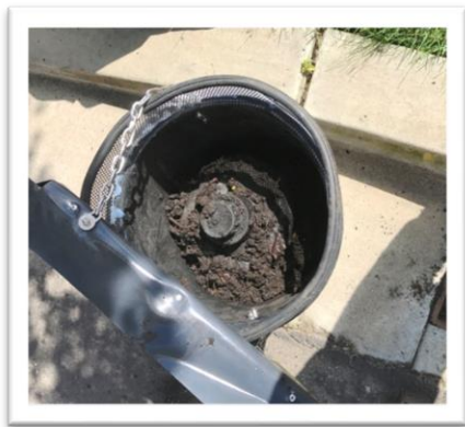
Image 11: Inspection and Cleaning of a side inlet with a Water Decontaminator Model #TCU-4. Leaves and sediment present and removed. Housing cleaned, sediment collected and disposed. Note special support frame. ( Deflector removed for visual purposes )
