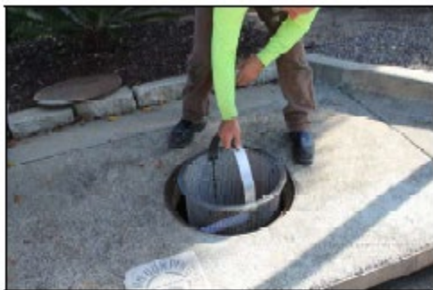
Figure 17 - Curb Inlet Filter Basket Being Installed.
