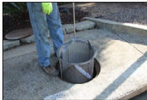
Figure 18 - Curb Inlet Filter Basket Being Installed.
