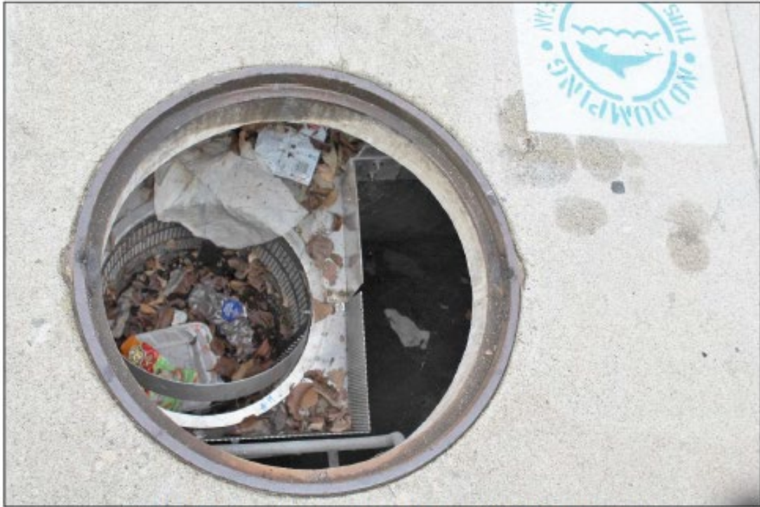
Figure 24 - View 1 of Catch Basin Bottom with Bio Clean® Curb Inlet Filter Installed
