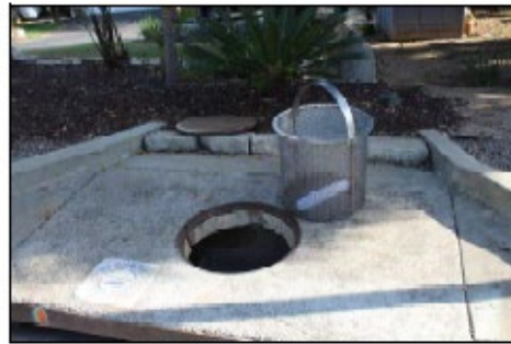
Figure 16 - Curb Inlet Filter Basket Being Installed.
