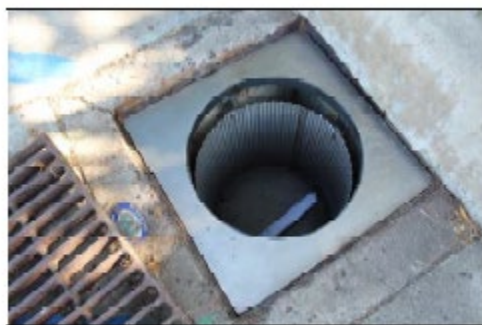
Figure 11 - Grate Inlet Filter (no access window) Installed.
