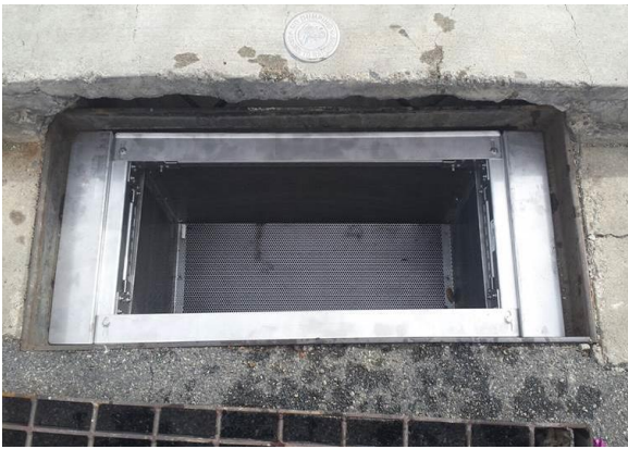
Photos 2 and 3: PURE FTC inserts shown during installation into a catch basin
