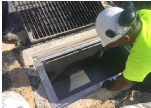
Photos 2 and 3: PURE FTC inserts shown during installation into a catch basin
