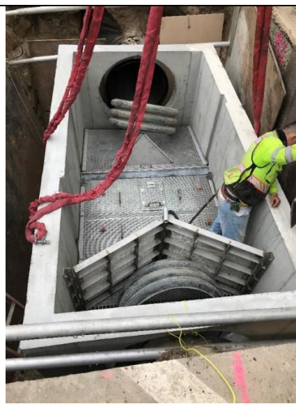
Figure 2 – Back view looking towards inlet
