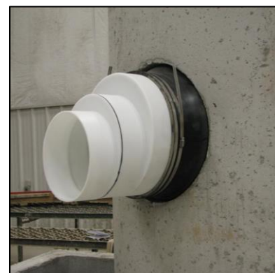
Figure 4 - Example Outlet Module Connection w/ Flexible Boot
