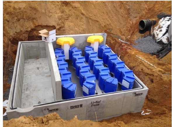
Figure 10 - Up-Flo® Vault w/ Double Array
