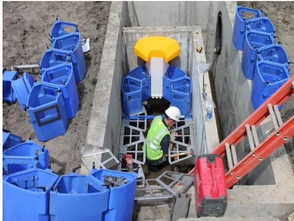
Figure 9 - Up-Flo® Vault w/ Single Array Module Install
