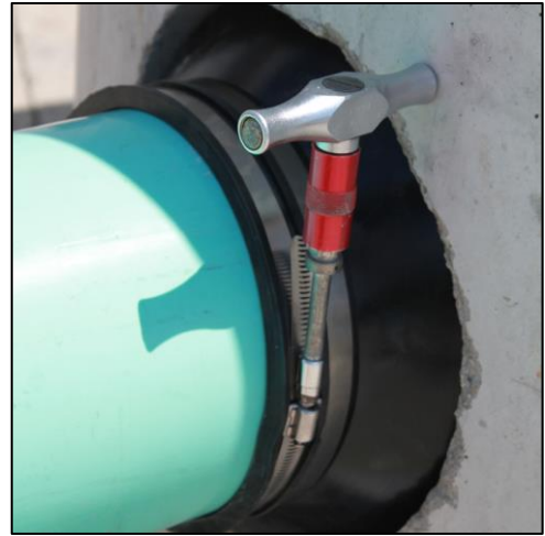
Figure 6 - Example Boot Connection to Vault
