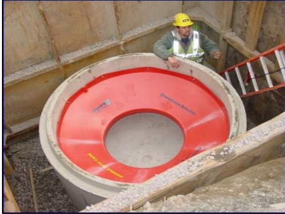
Figure 3 – Benching Skirt Install and Placement
