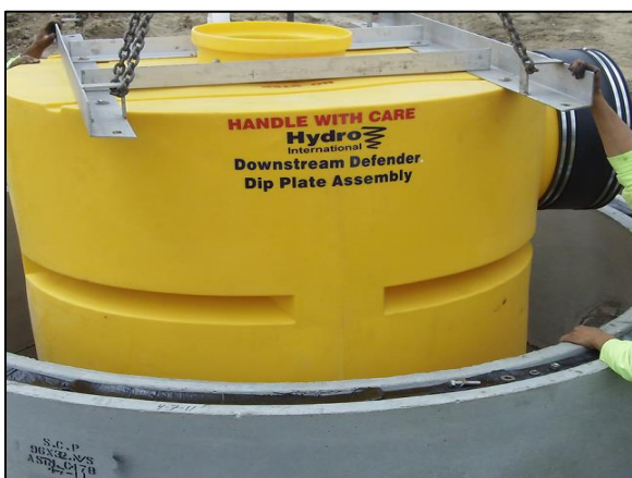
Figure 5 – Close-up Side View of Dip Plate
