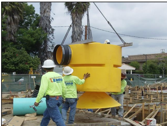
Figure 4 - Defender® Dip Plate and Cone ready for Install
