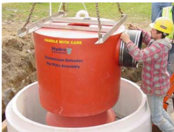
Figure 7 – Dip-Plate Assembly Insertion Into Manhole
