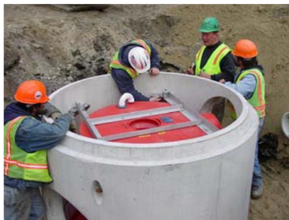
Figure 8 - Dip-Plate Assembly Mounting to Manhole
