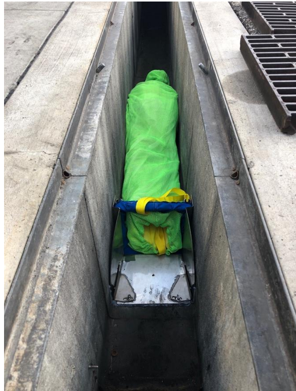
Figure 2 - Marine terminal install – looking downstream
