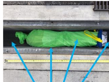
Vector control placement areas: upstream, within, under or downstream of Mundus Bag™
