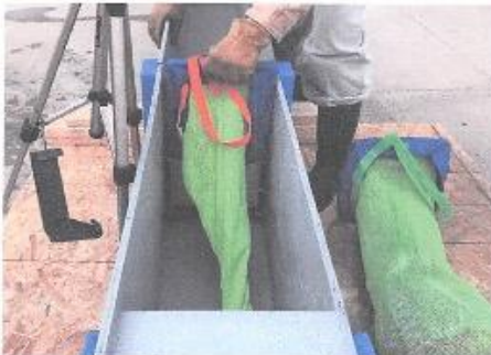
Removal of the Mundus Bag for maintenance or service
