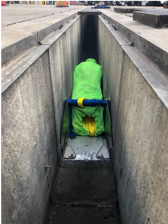
Figure 1 – Marine terminal install – looking downstream
