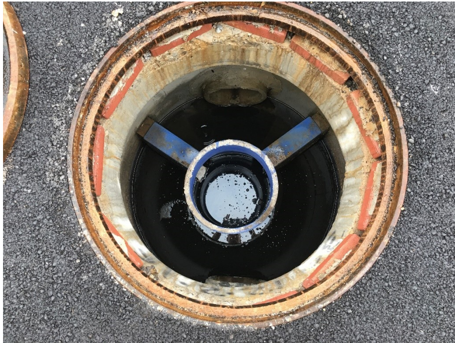
Figure 5 - View from Manhole Access Point
