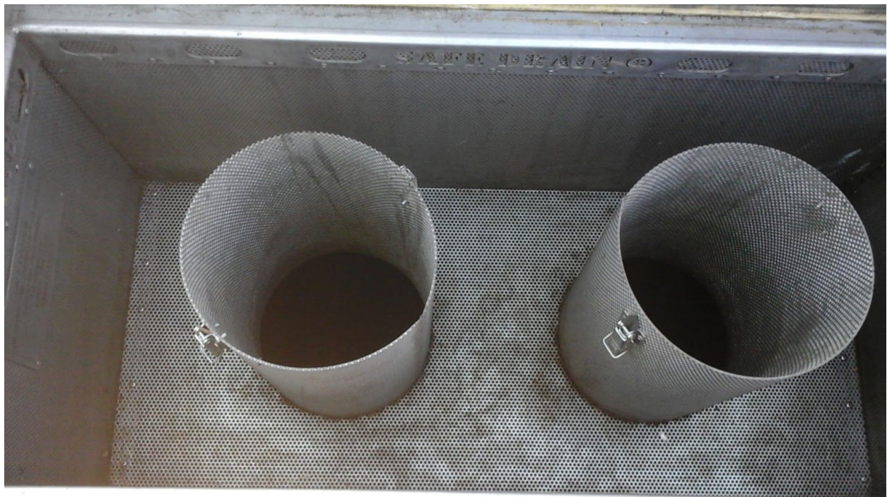
FIG. 4 - Modesto Full Trash Capture Device - Dual Stove Pipe Overflow and Vector Control Access Ports - All Surfaces Perforated - 3.175 mm - No Cover Cap
