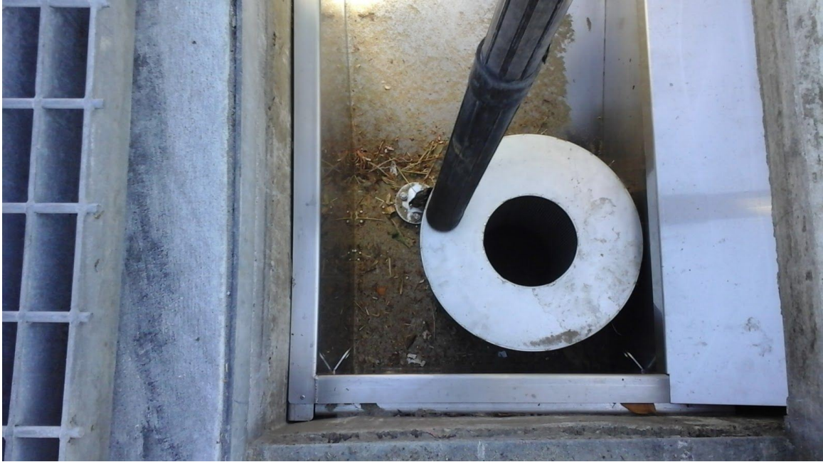
FIG. 7 - Santa Cruz Sand, Silt and Full Trash Capture Device - Cleaned
