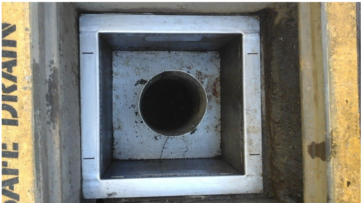
FIG. 2 - Modesto Full Trash Capture Device - Single Overflow Stove Pipe and Vector Access Port - All Surfaces Perforated - Cleaned Out
