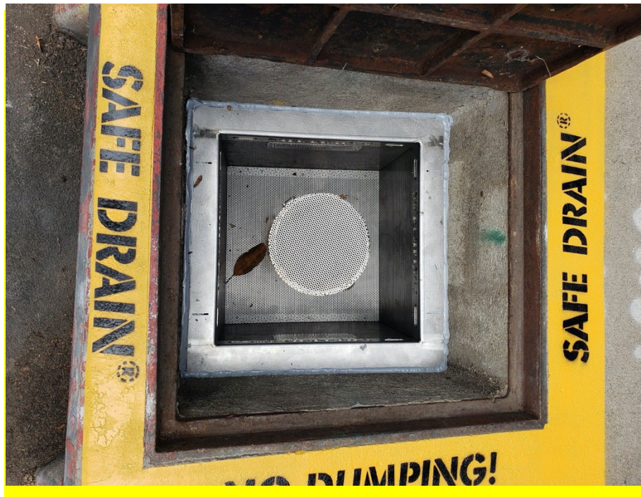
FIG. 4 - Modesto Full Trash Capture Device - Dual Stove Pipe Overflow and Vector Control Access Ports - All Surfaces Perforated - 3.175 mm - No Cover Cap
