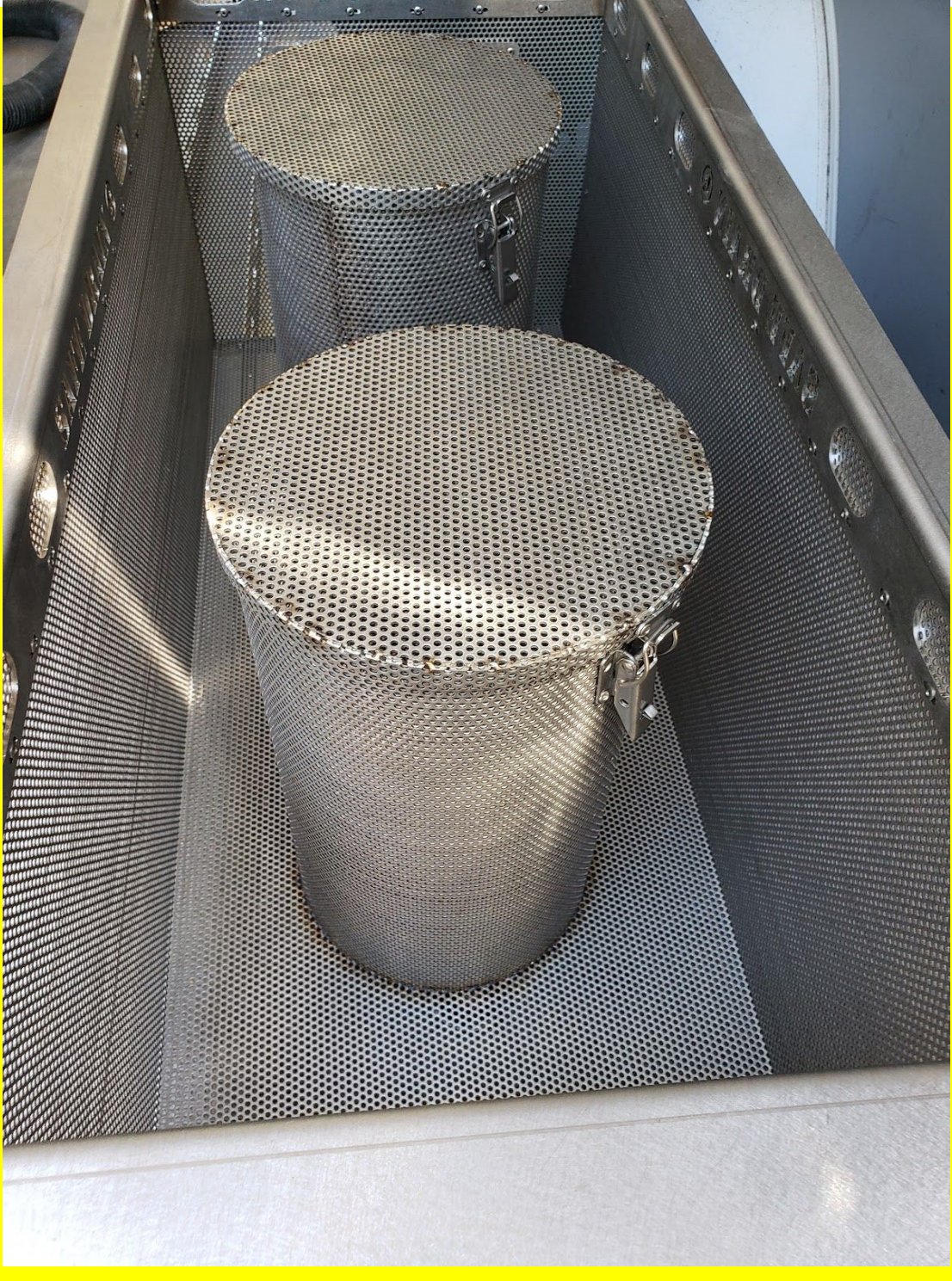
FIG. 5 - Modesto Full Trash Capture Device - Dual Stove Pipe Overflow and Vector Control Access Ports - All Surfaces Perforated - 3.175 mm - Cover Caps Installed
