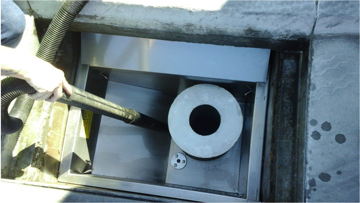
FIG. 7 - Santa Cruz Sand, Silt and Full Trash Capture Device - Cleaned
