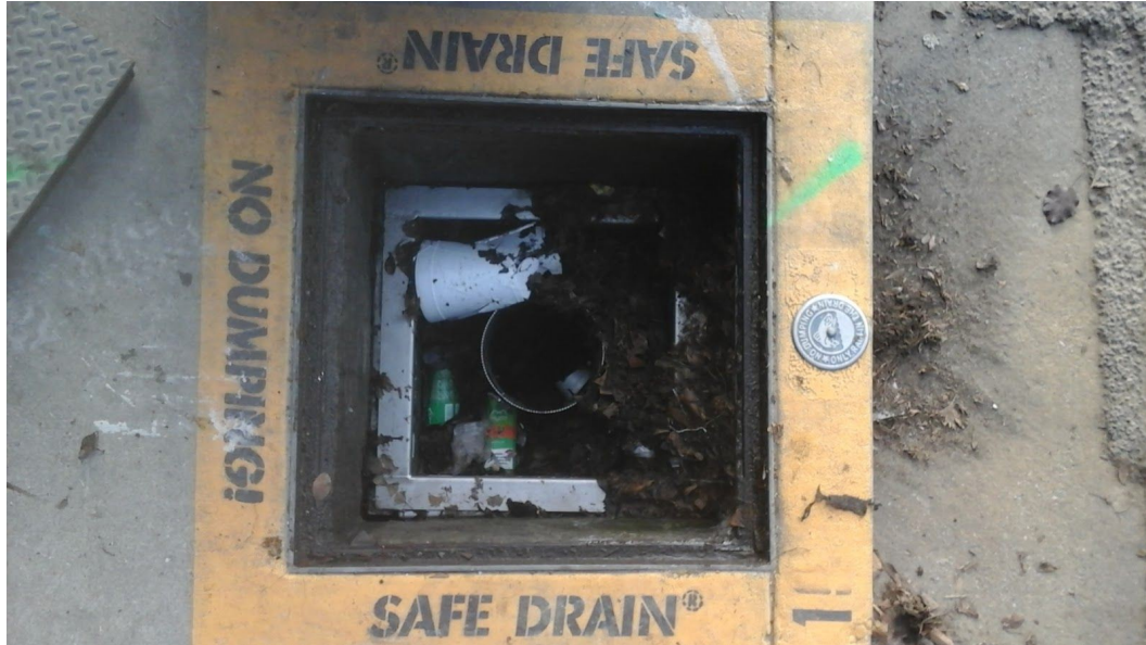
FIG. 2 - Modesto Full Trash Capture Device - Single Overflow Stove Pipe and Vector Access Port - All Surfaces Perforated - Cleaned Out
