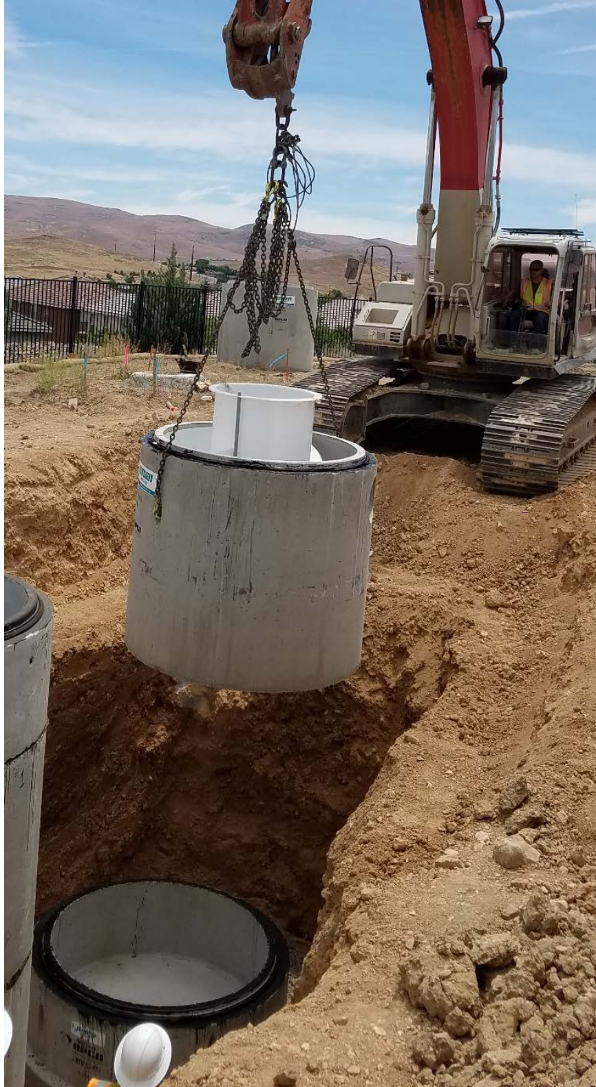
Figure 12. Separation Chamber of 1.1-cfs Capacity JDS60-2424 Unit Set in the Field on Top of Sump. The JDS60-2424 is Handled and Installed as Typical 60-in ID Precast Manhole Riser Piece.
