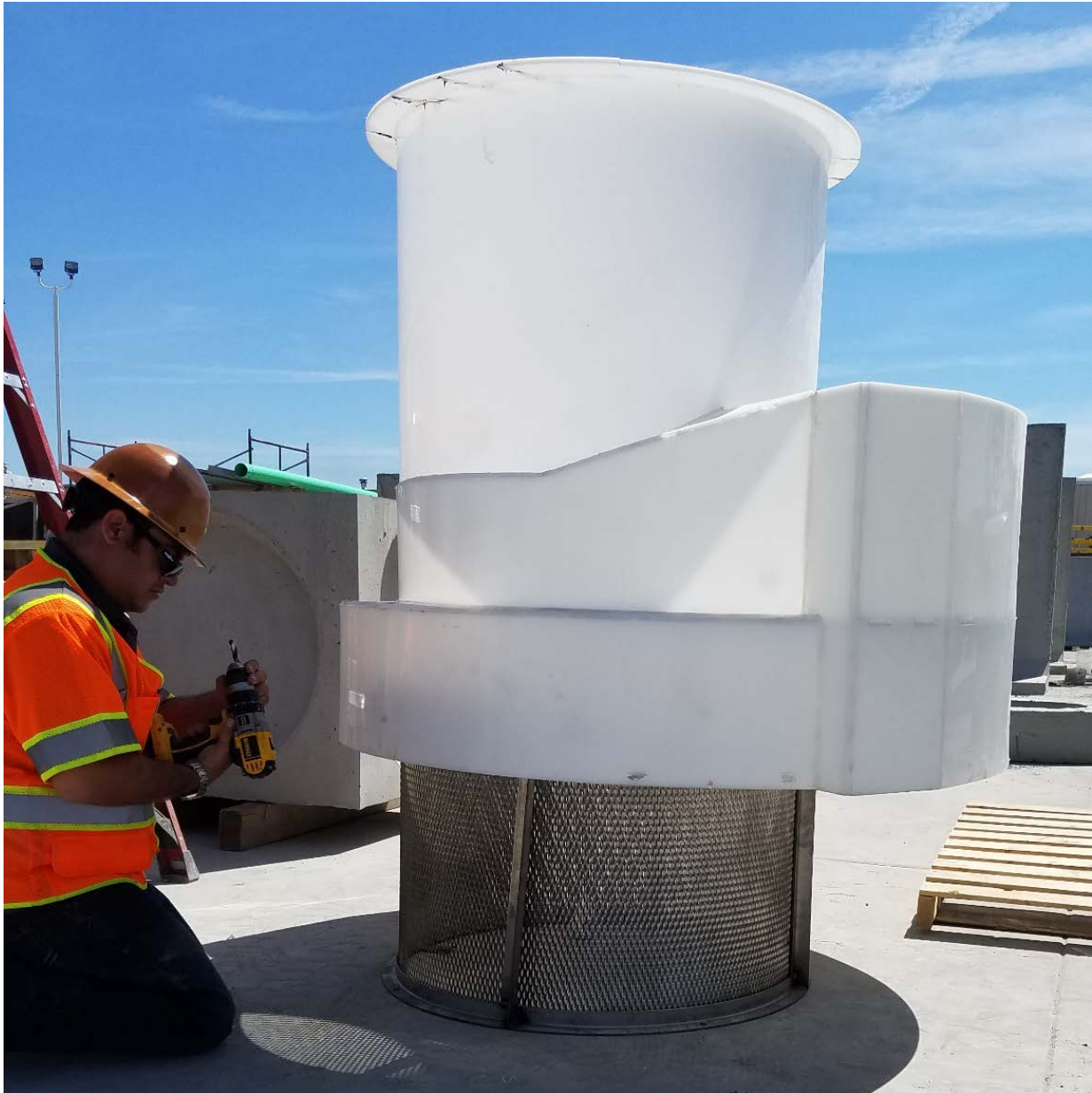
Figure 9. Assembly of SS Screen to HDPE Inlet for 1.1-cfs Capacity Inline JDS60-2424 .
