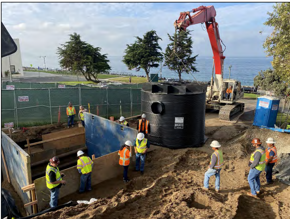
Installation of Aqua-Swirl® Trash Capture Model AS-12s, Redondo Beach, CA.
