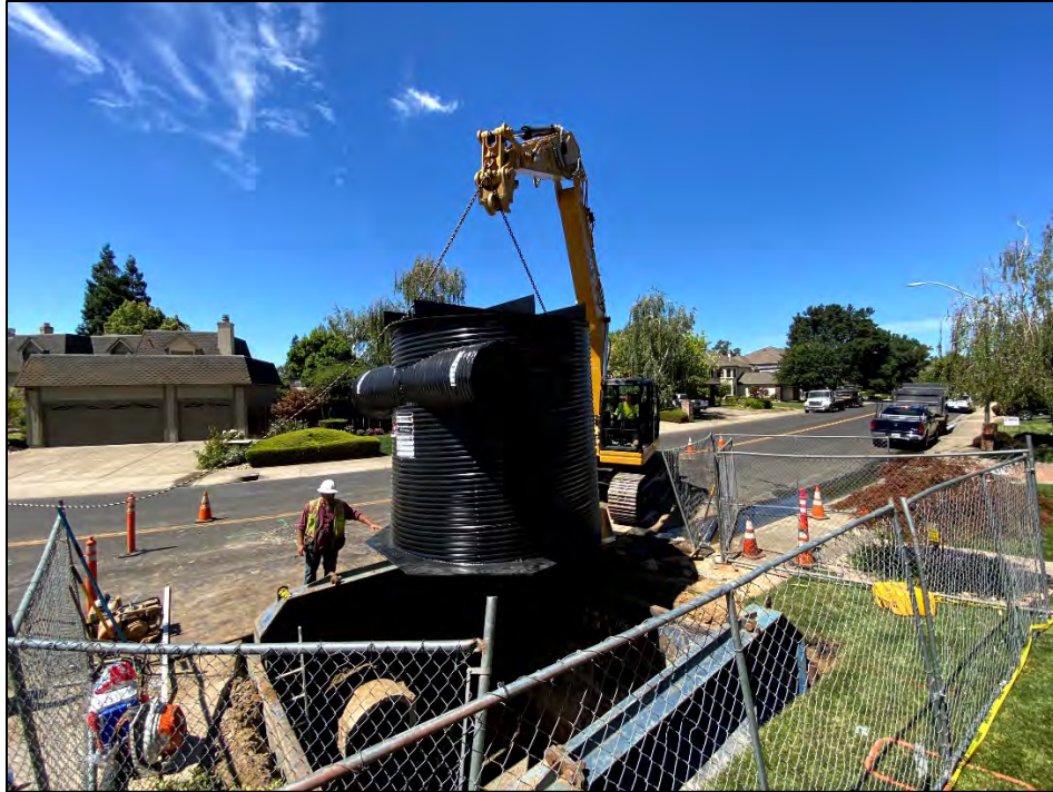
Installation of Aqua-Swirl® Trash Capture Model AS-10s, Lodi, CA.
