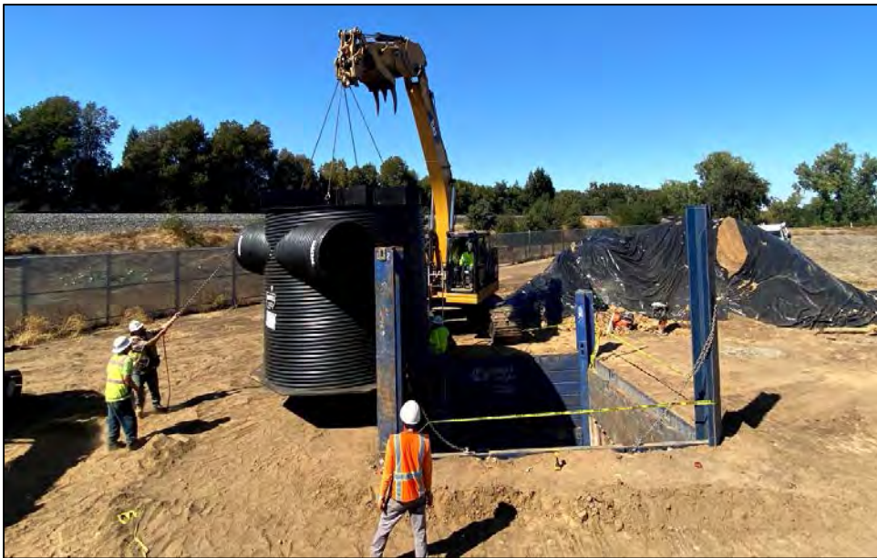
Installation of Aqua-Swirl® Trash Capture Model AS-11s, Lodi, CA.
