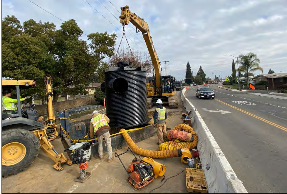
Installation of Aqua-Swirl® Trash Capture Model AS-8s, Lodi, CA.
