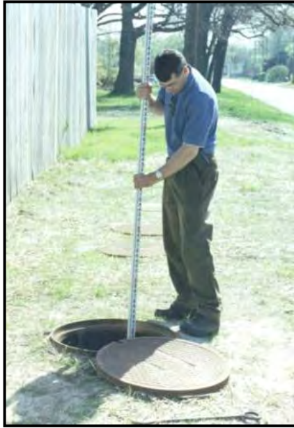
Sediment inspection using a stadia rod
