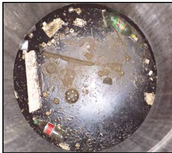
Floatable debris in the Aqua-Swirl ®
