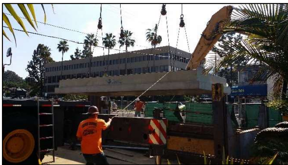
Figure 6 - DSBB Base Slab Installation
