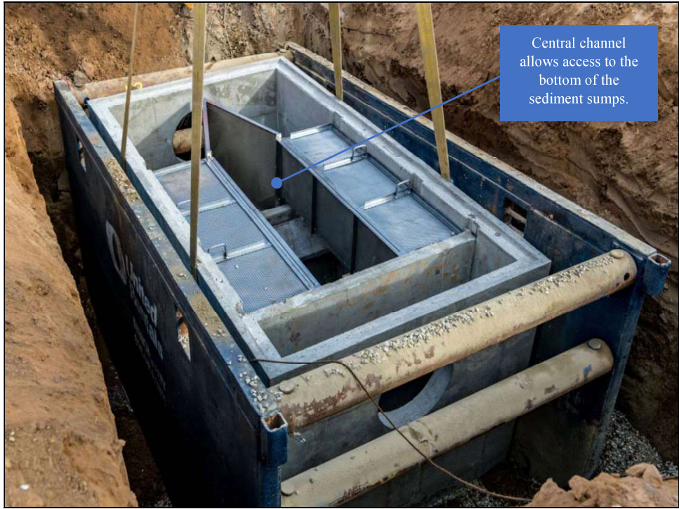
Figure 18 - Installation of DSB Showing Central Access Maintenance Channel
