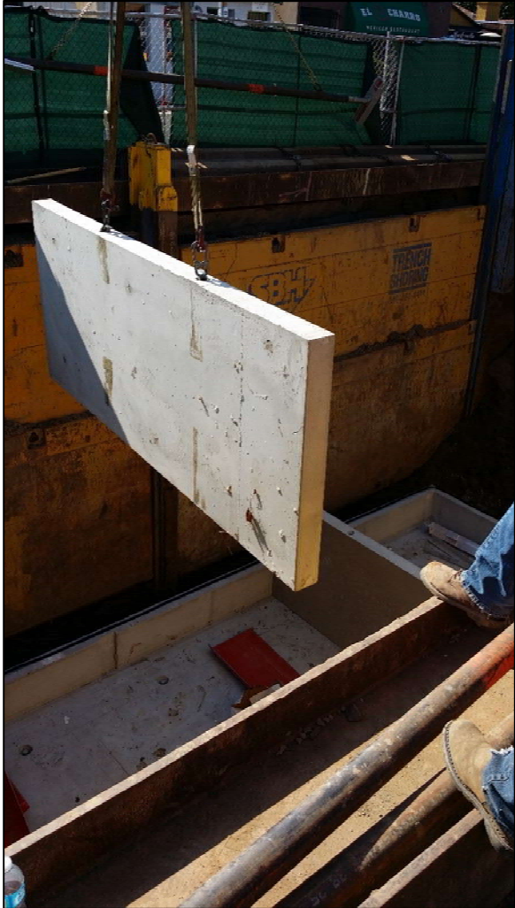
Figure 8 - DSBB Baffle Wall Installation
