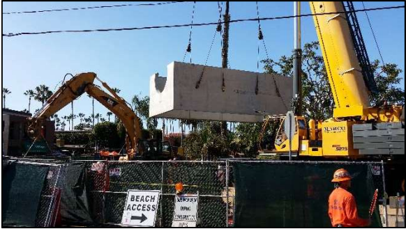
Figure 10 - DSBB Treatment Section Installation
