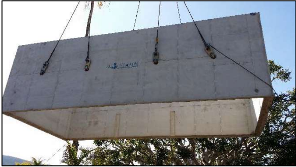
Figure 9 - DSBB Treatment Section Installation
