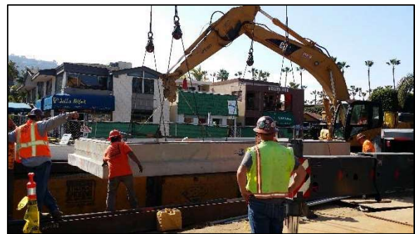
Figure 7 - DSBB Base Slab Installation
