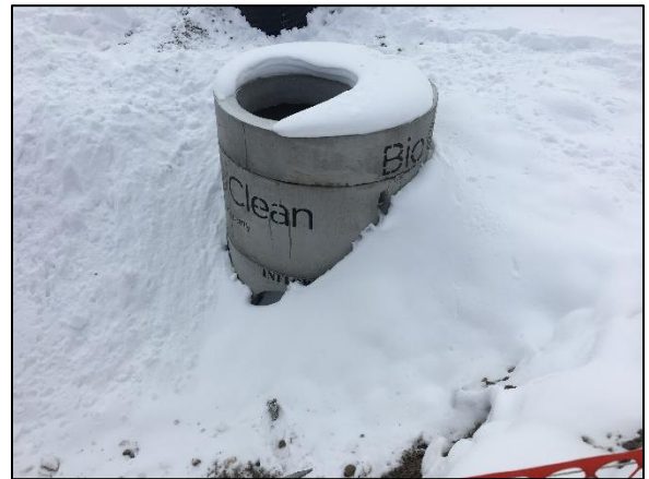
Figure 10 – DSD Installed Waiting for Backfill
