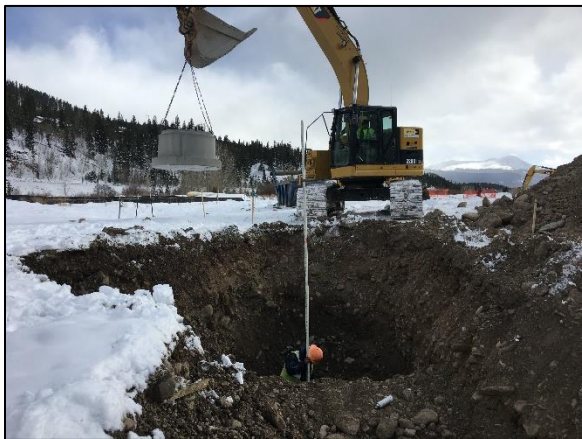
Figure 6 – DSD Sump Section Offload and Set
