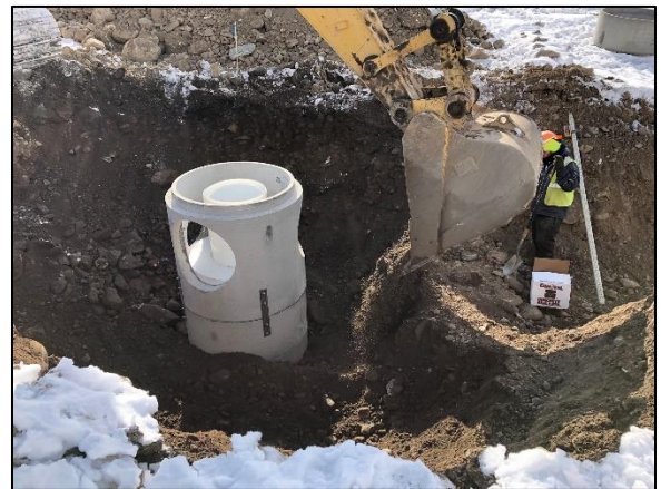
Figure 9 – DSD Treatment Section Placed
