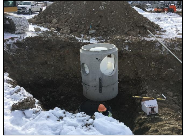
Figure 8 – DSD Treatment Section Offload
