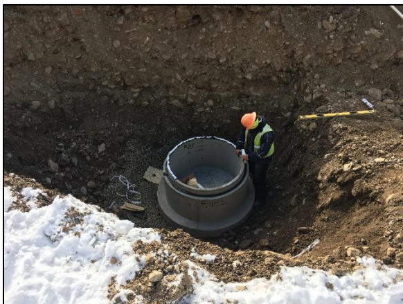
Figure 7 – DSD Sump Section Placed
