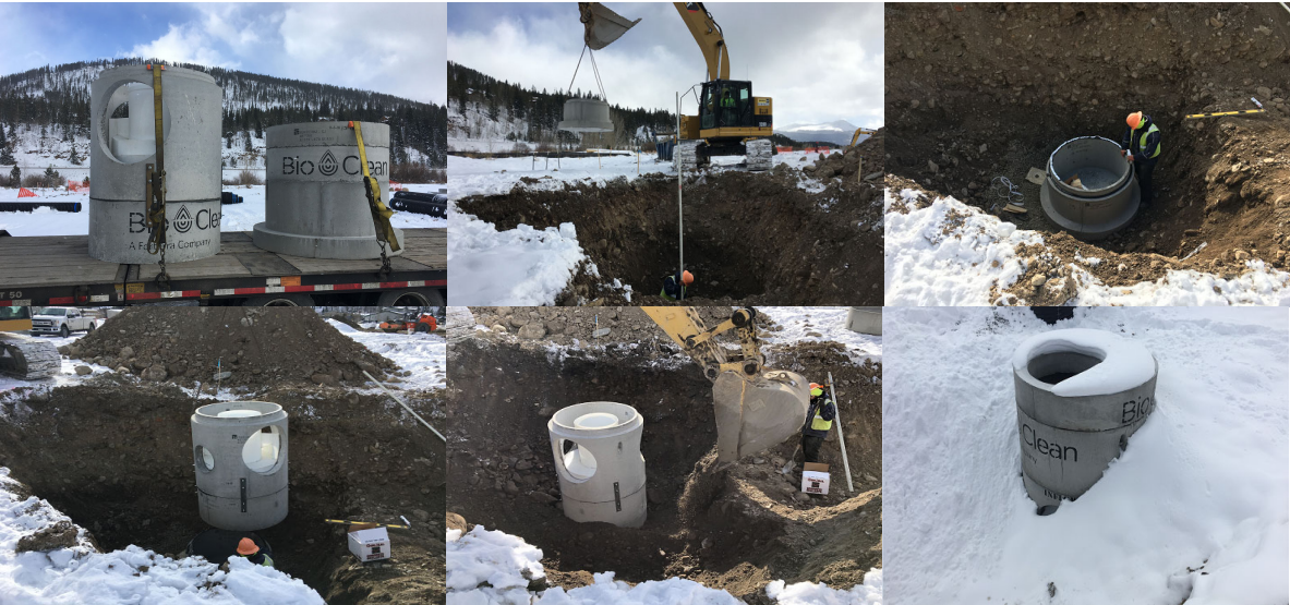
Set the access risers (if applicable) to bring the manhole frame and covers up to finish surface elevation per the approved drawings and plans.
