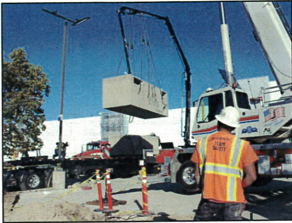
Figure 6 – Modular Wetlands® Offload From Truck
