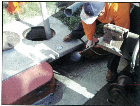
Figure 17 - Maintenance of Modular Wetlands® System
