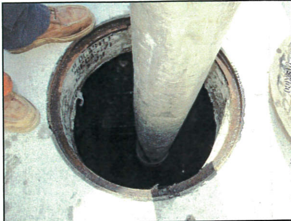
Figure 18 - Maintenance of Modular Wetlands® System
