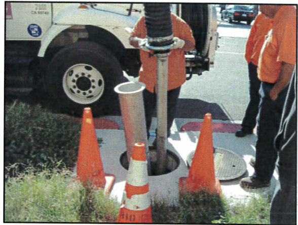
Figure 16 - Maintenance of Modular Wetlands® System
