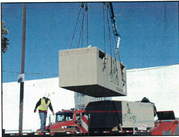
Figure 7 - Modular Wetlands® Offload From Truck
