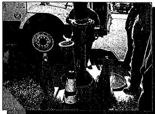
Insertion of vacuum hose into separation chamber.
