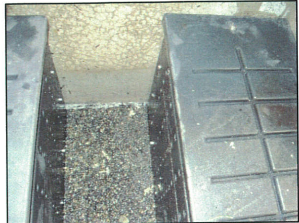
Figure 20 - Pre-Treatment Chamber Post-Maintenance
