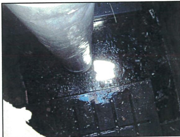
Figure 19 - Maintenance of Modular Wetlands® System
