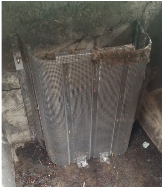
Figure 4 – Connector Pipe Screen Installed (U-Shaped)
