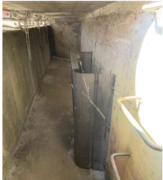
Figure 5 – Connector Pipe Screen Installed (U-Shaped)
