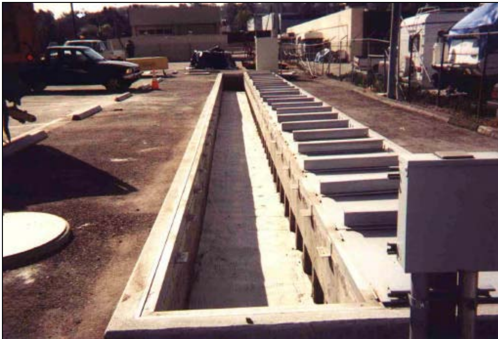
Figure 2-4 Escondido MS Delaware Sand Filter
