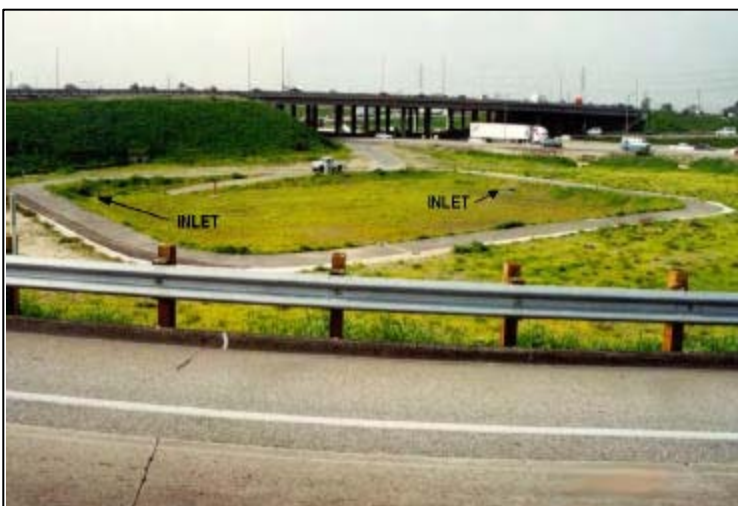
Figure 5-2 I-605/SR-91 Infiltration Basin
