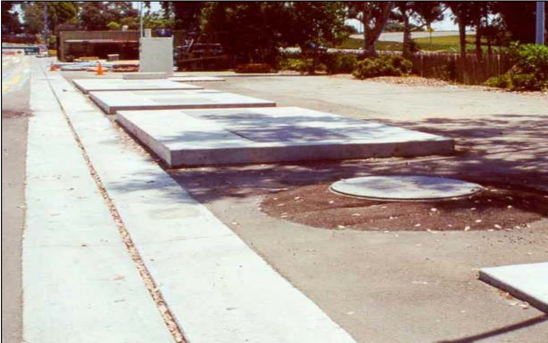
Figure 9-2 Surface View at Kearny Mesa
