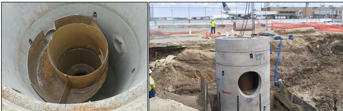
Figure 6 - Typical inline installation
