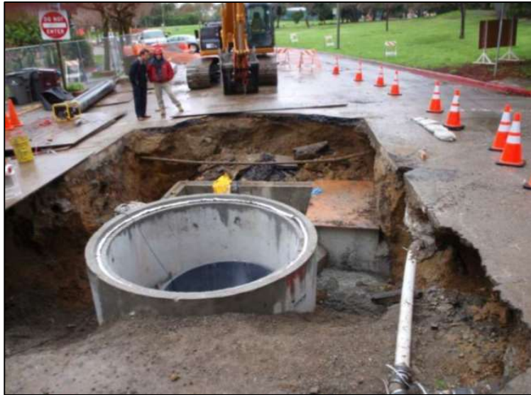
Figure 7 - Typical offline CDS installation
