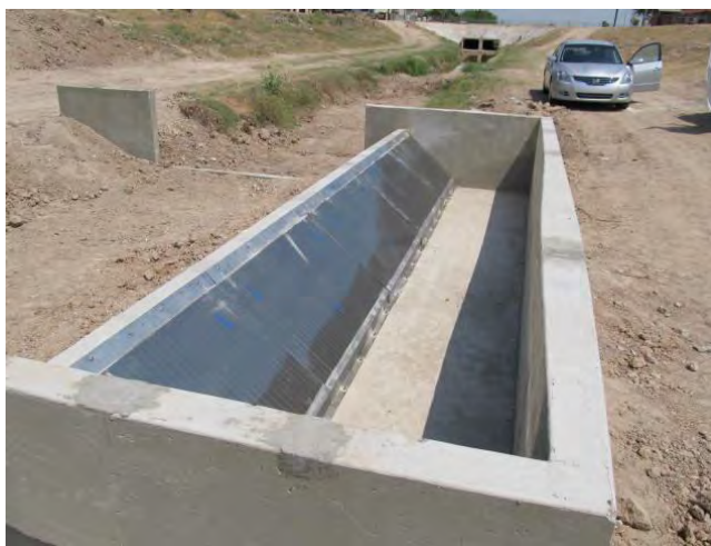
Figure 2. McAuliffe RDF Coanda Screen
