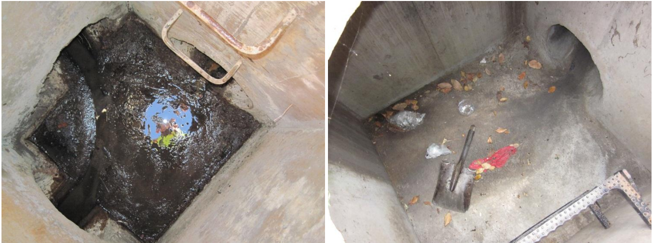
Figure 29. Catch basin interiors, showing deep and shallow sumps in Tecolote and San Ysidro.
