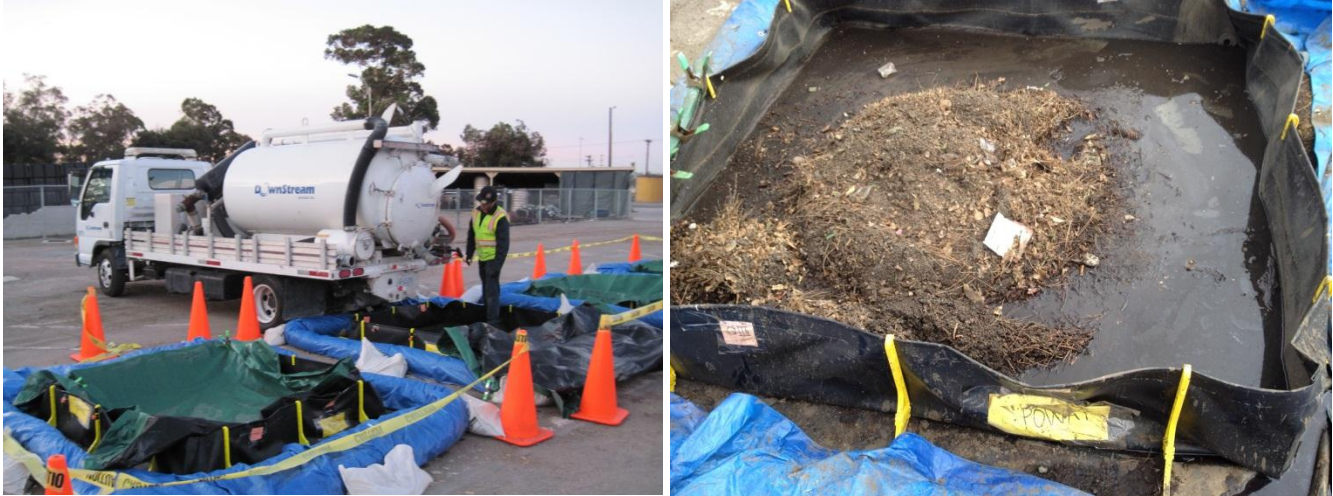
Figure 8. Delivery of materials to the containment berms for storing and drying before sampling and analysis.
