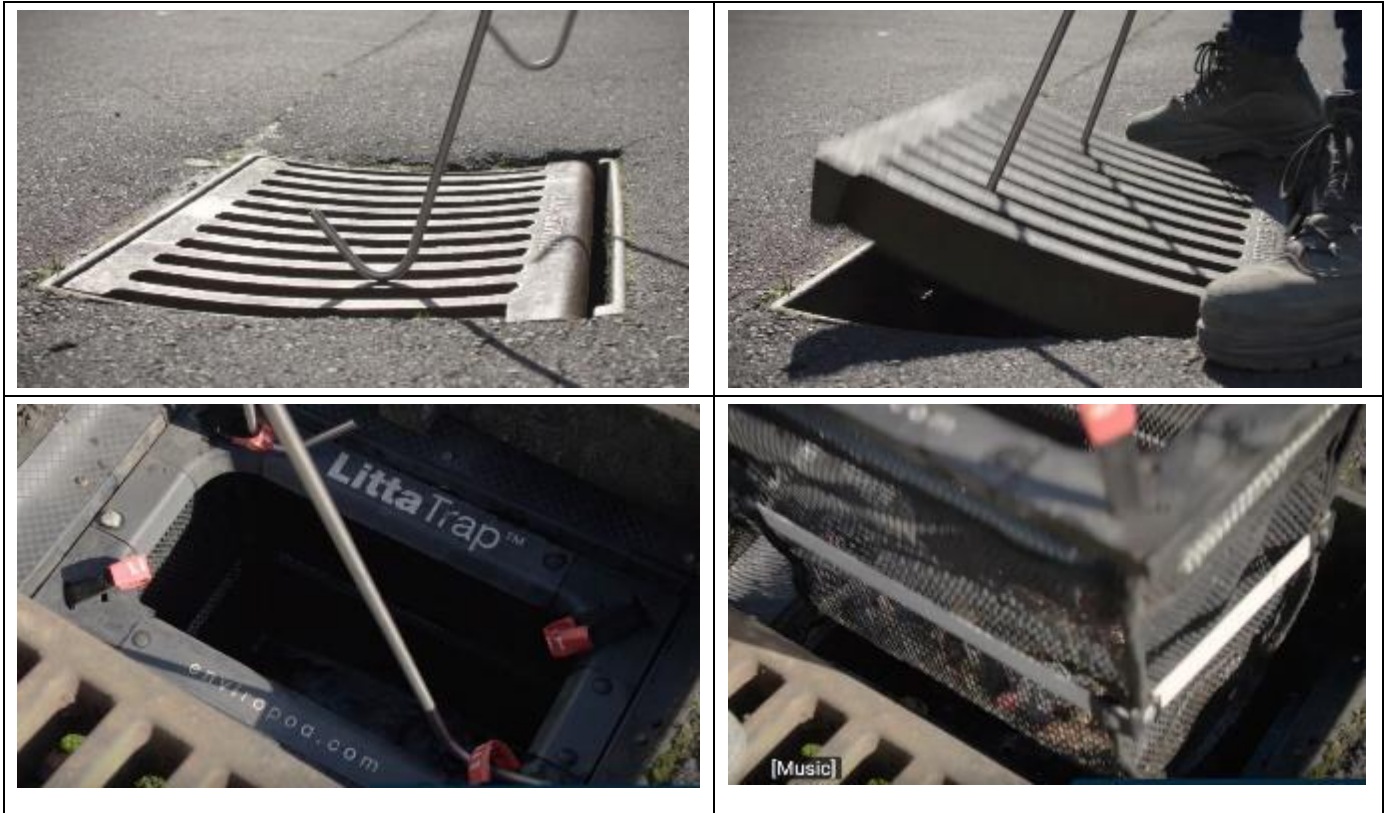
Figure 12: Example of Post Installation and Maintenance
