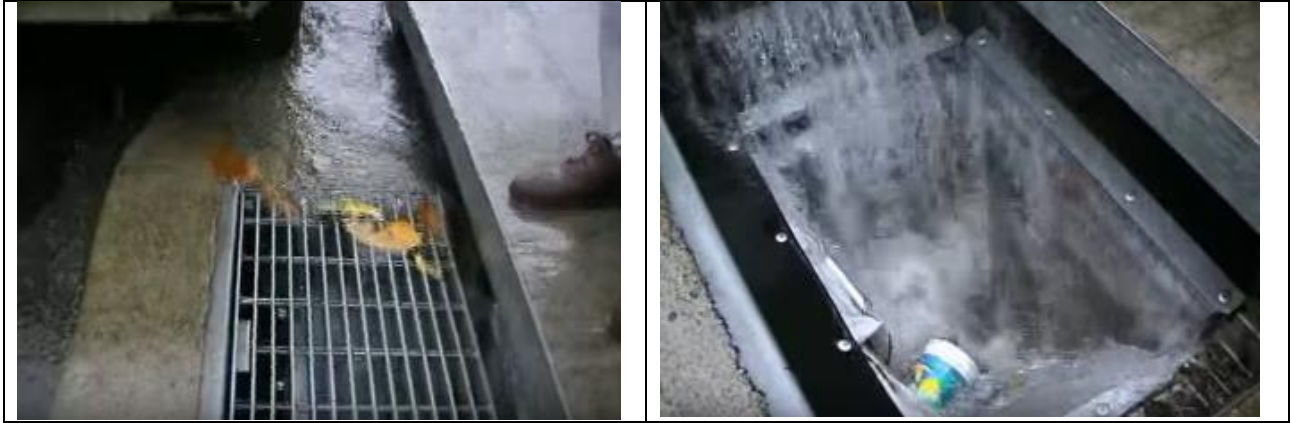
Figure 11: Post Installation Operation
