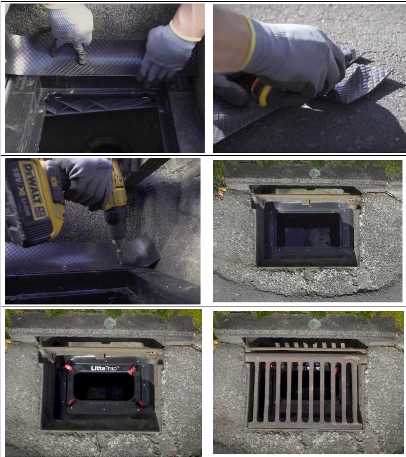
Figure 10: Installation Process Part 2
