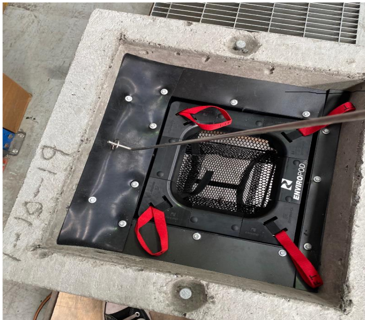
Figure 15: Enviropod® LittaTrap™ FC with Vector Inspection seal in closed position.
