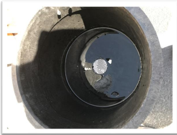
Image 14: 3/16" Screen at 3 inch diameter opening.
