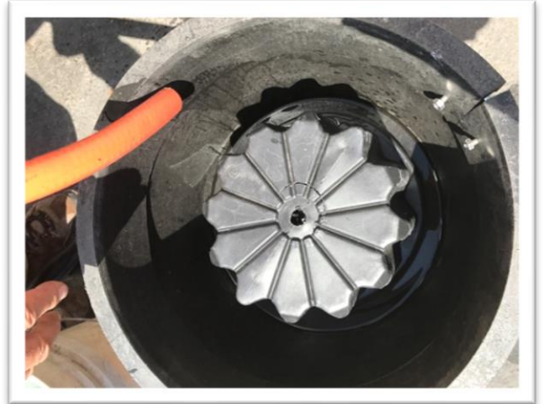
Image 15: Energy Dissipater added to top of opening to avoid jet flow.
