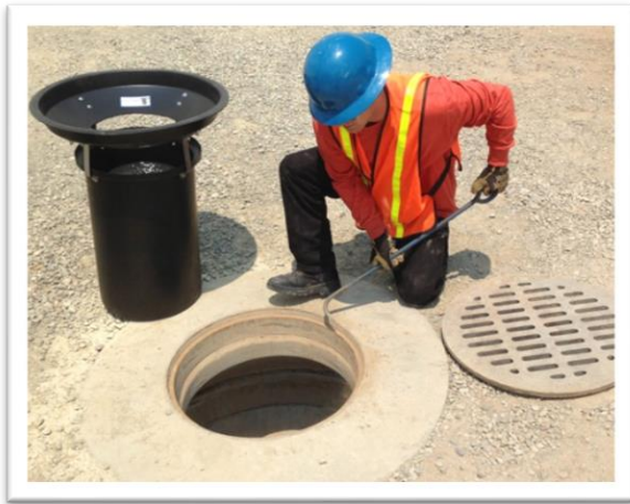
Image 10: Installing unit, checking lip and removing rust.
