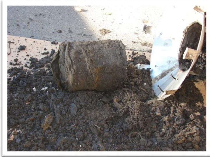
Image 12: Decomposed leaves after the Fall season and leaf drop. This street was not properly street swept and all the leaves went down the catch basin and into the unit. This unit has a SS deflector.
