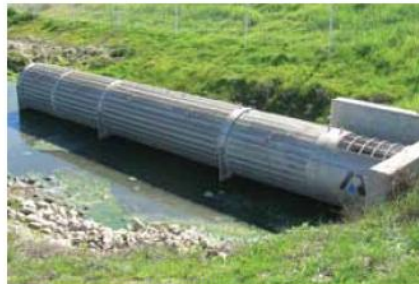
End of pipe installation for detention ponds.
