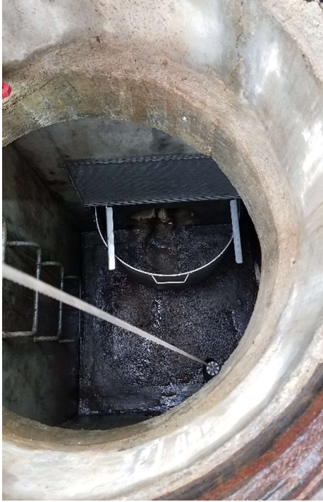
Figure 1. City of Poway - Location 1; 1 month post installation.
