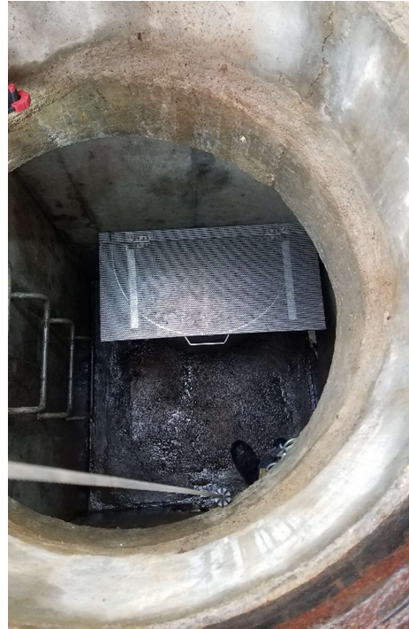
Figure 2. City of Poway - Location 1; 1 month post installation.
