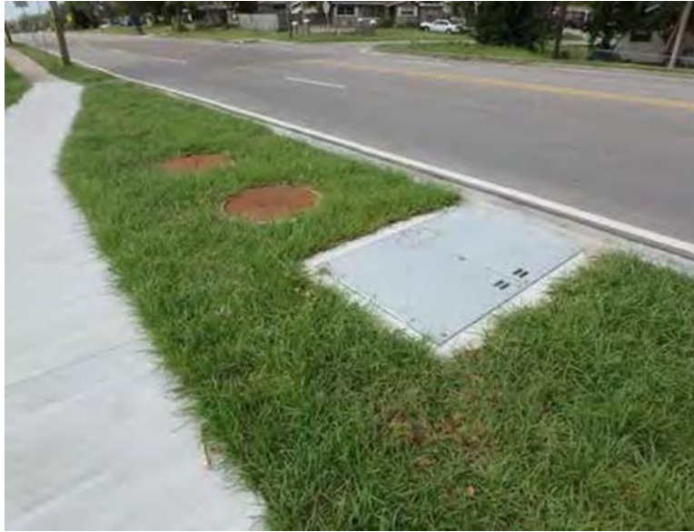
Finished installation. Two manhole castings shown provide access to the vault.
